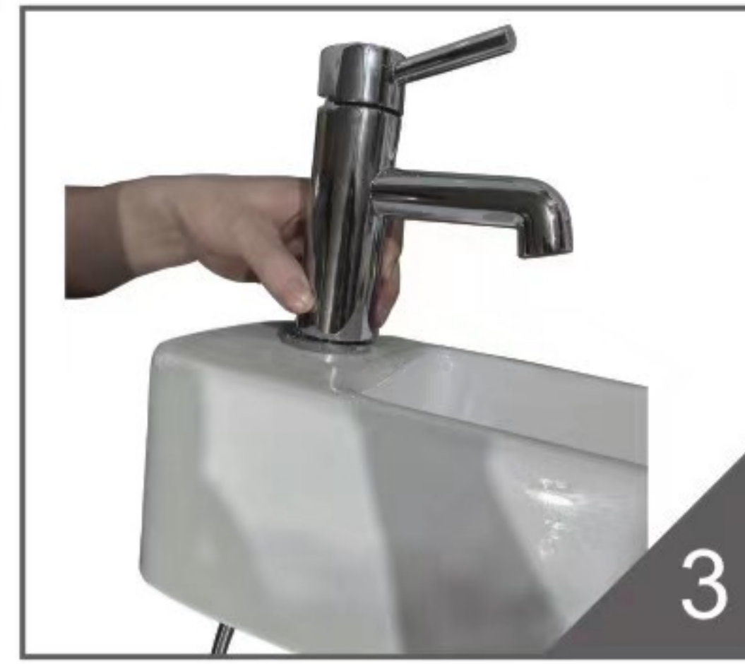
2-5: Install the faucet on the basin and connect the inlet pipe.
