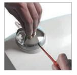
Set the control lever to mid-blend (12 o'clock) position prior to removing the three fixing screws and withdrawing the lever. Remove the fixing screw from the top of the Aquastream Thermo casing and pull the front cover away from the unit.
